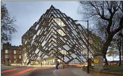
DIAMOND CENTRE, MAIN VENUE
